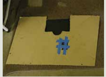
#22. A slot will need to be cut in the floorboard to accommodate the Mitchell shifting lever. Make a cardboard template to accurately locate the positioning of the slot.
